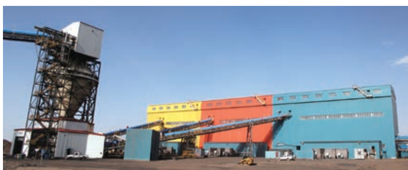
CHPP with 3 modules completed
